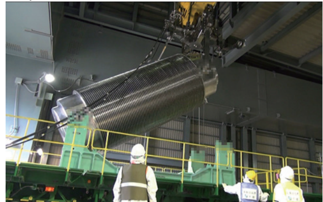
Loading the transfer vessel onto a trailer
